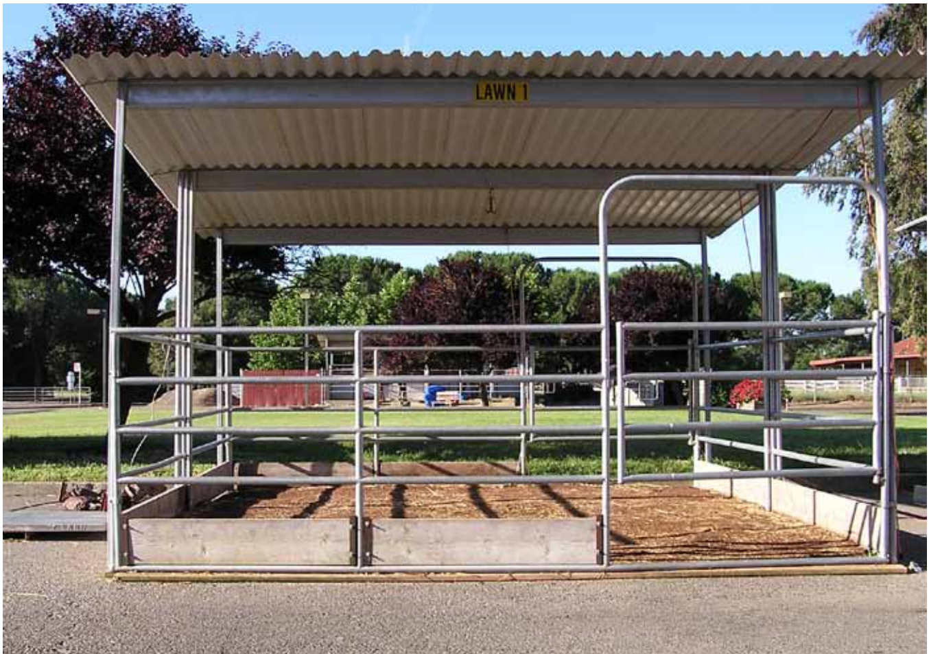
This is the type of portable structure that can be used to create an isolation unit at an equine facility or event.
